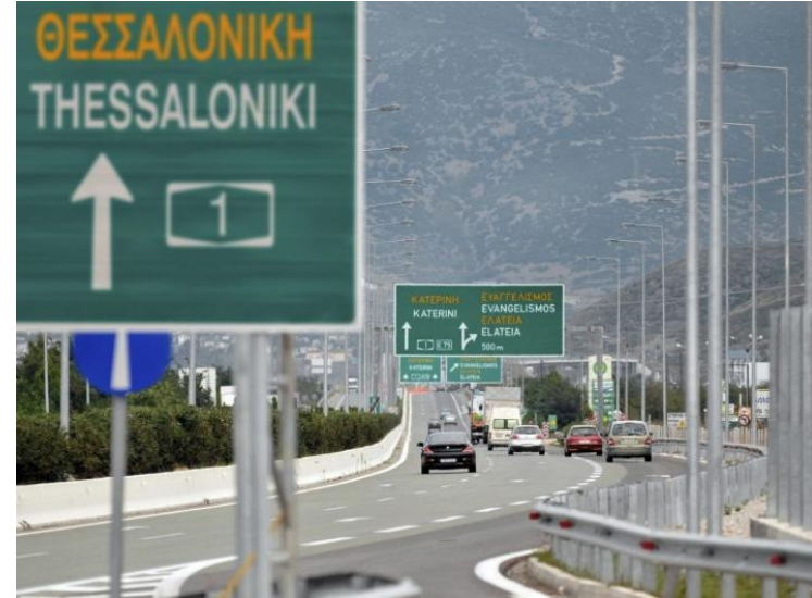
Maliakos-Kleidi motorway, Greece Investment volume: 1.1 Mld.€
