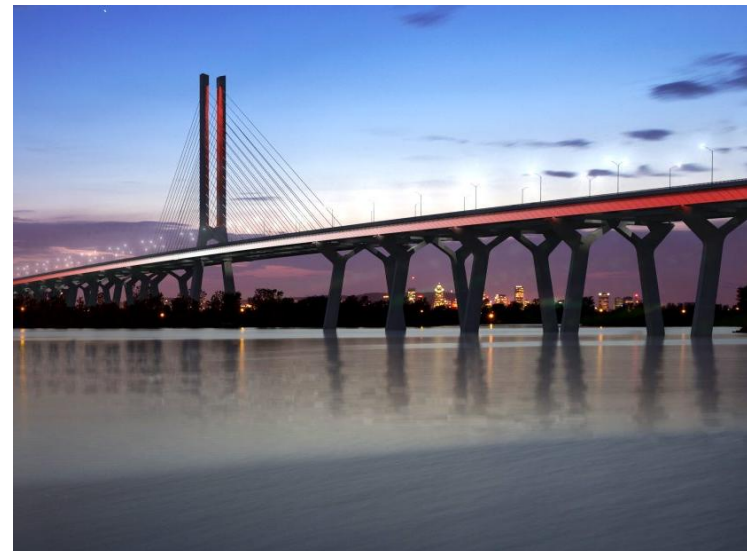
New Champlain Bridge Montreal, Canada CAPEX: 1.6 Mld.€
